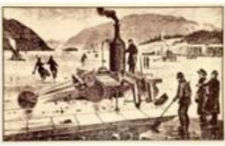
Jager's steam-driven machine for sawing ice into blocks (1833)
